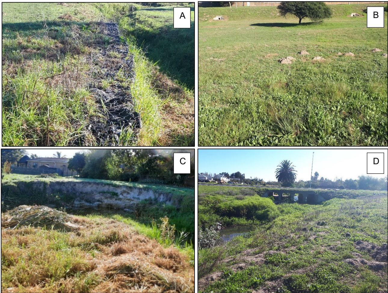
Figure 5.3 Photos taken while conducting wetland assessments at 2AU1 on 12/05/2021. A) Sections of the river channel stabilised with gabions, B) Stormwater drains emptied into the wetland and its surrounds, with non-native weed overgrowth, C) Erosion of the river banks in the upper reaches of the wetland, and D) Channelisation of the headwaters of the wetland.
