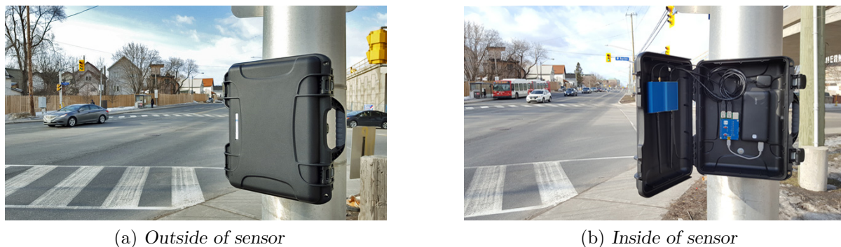
FIGURE 1.2: A SMATS Wi-Fi and Bluetooth sensor attached to a lamp post [147].
