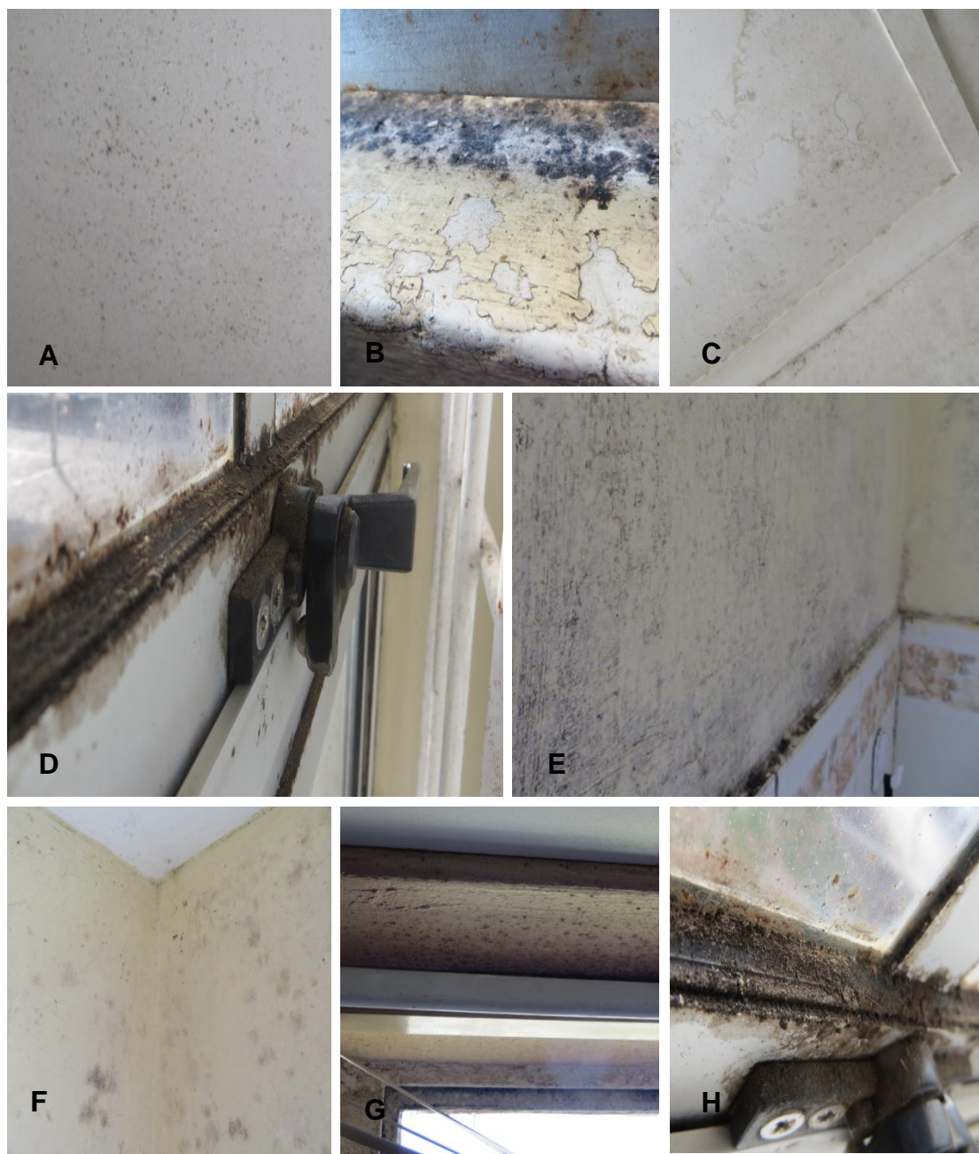
Figure 2.1. Cladosporium contamination from different parts of indoor environments. A and C. ceiling boards. B and G. window seals. D and H. window frames. E and F. Walls.
