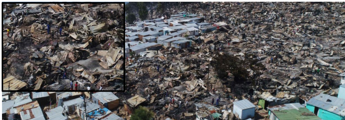
Fig. 4-6: Aerial image of Imizamo Yethu after the 2017 fire (Image used courtesy of Bruce Sutherland, City of Cape Town)
