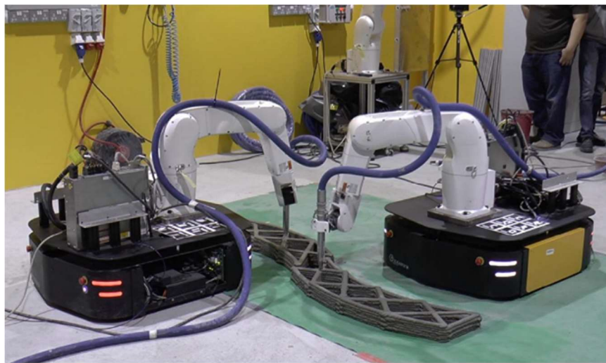
Fig. 2.7: Concurrent 3D concrete printing concept demonstrated by [43].
