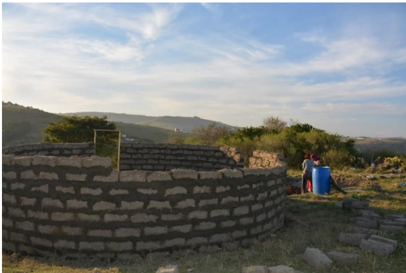
Figure 6: Building first rondavel for the cultural centre using self-made bricks.
