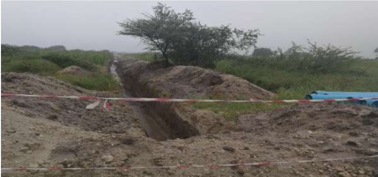
Figure 4.15: A CRIDF funded water pipeline in Mayana is intended to supply water to small-scale farmers in Mayana.
