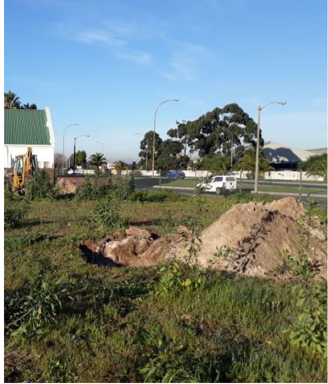
Figure 3-4: Stockpiled sand at Bellville South
