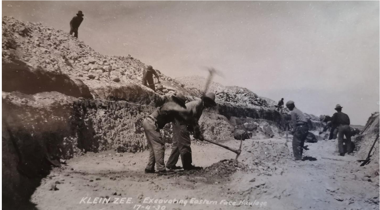
KLEIN ZEE. Excavating Eastern Face Haulage 17-4-30 “KLEINZEE. Excavating Eastern Face Haulage 17-4-30”
