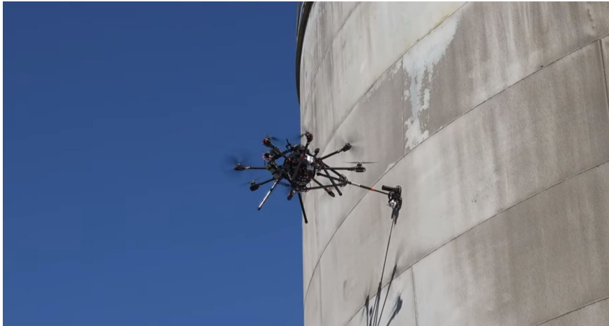
Figure 1.3: Multirotor inspecting a wall.
