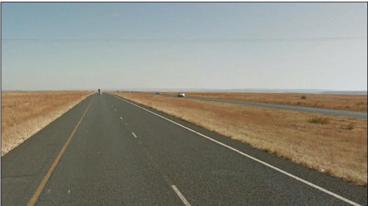
Figure 4-13: N4 Section 2f between Bossemanskraal and the Gauteng/Mpumalanga Provincial Boundary (Source: Google Street view)
