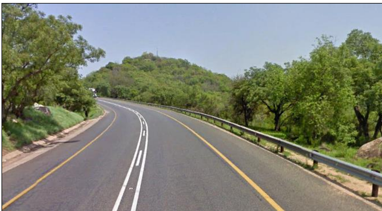
Figure 4-20: N4 Section 9, between Karino and Mara (Source: Google Street view)
