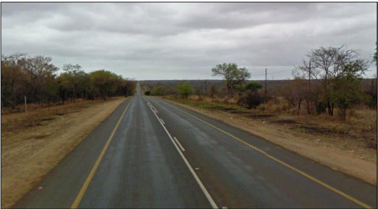
Figure 4-23: N4 Section 15A Hectorspruit to Komatipoort (Source: Google Street view)
