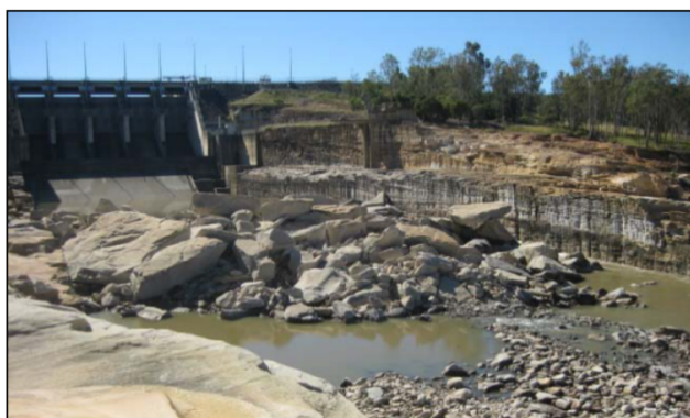
(b) Downstream scouring
