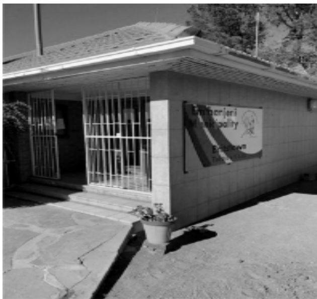
Figure 6.4: Britstown municipal offices
