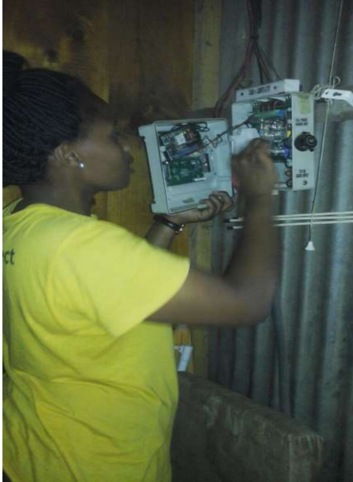
Figure 4.3: An iShack agent conducting maintenance checks on the Specialised Solar System
