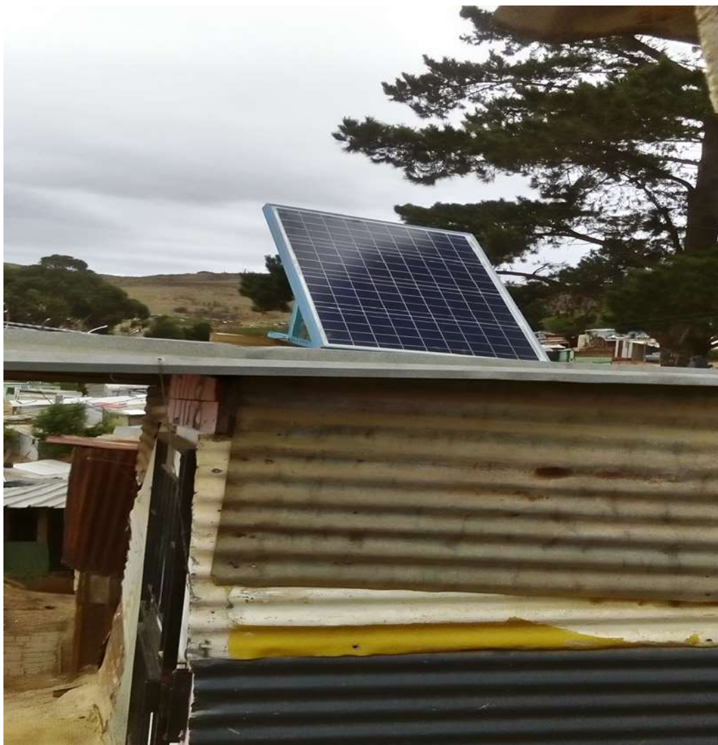
Figure 6: B. Box solar panel installed at a 50-degrees angle on top of a shack
