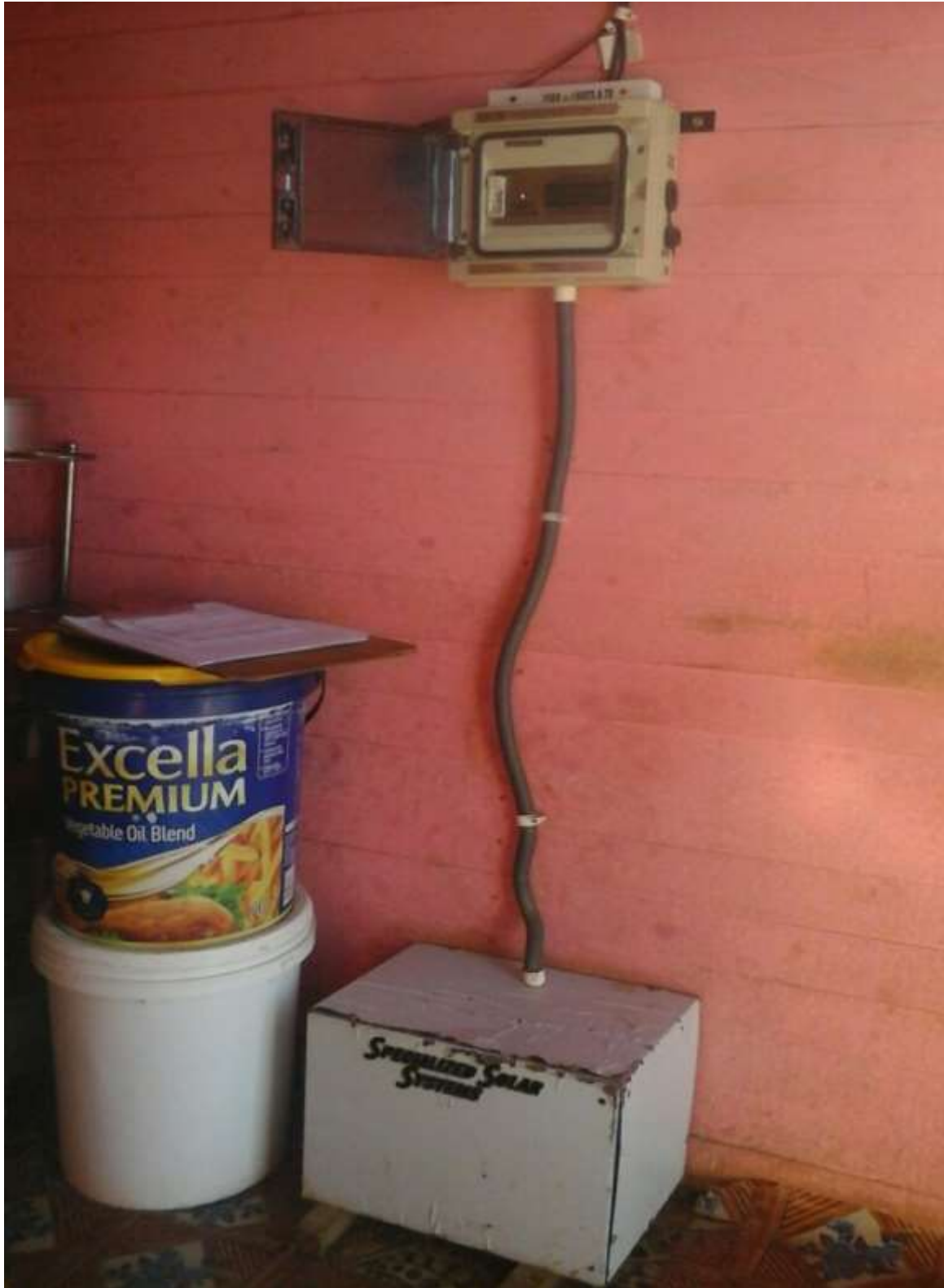
Figure 2: Installed Specialised Solar System
