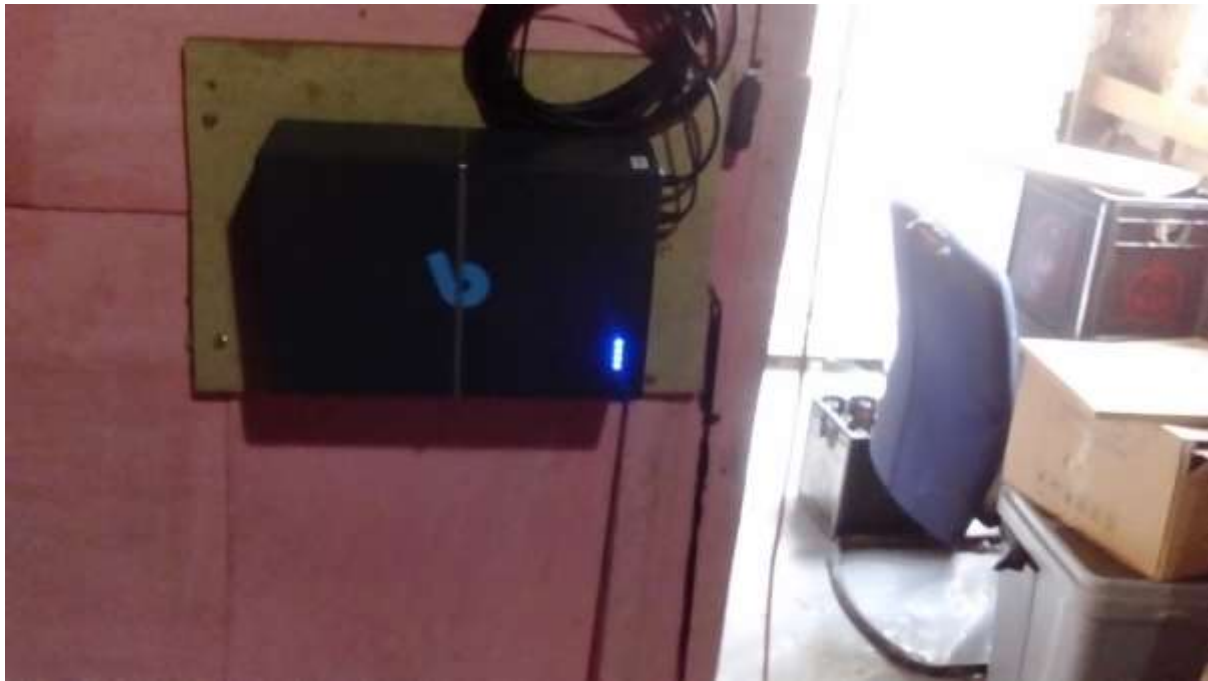
Figure 4: Installed B. Box solar system box
