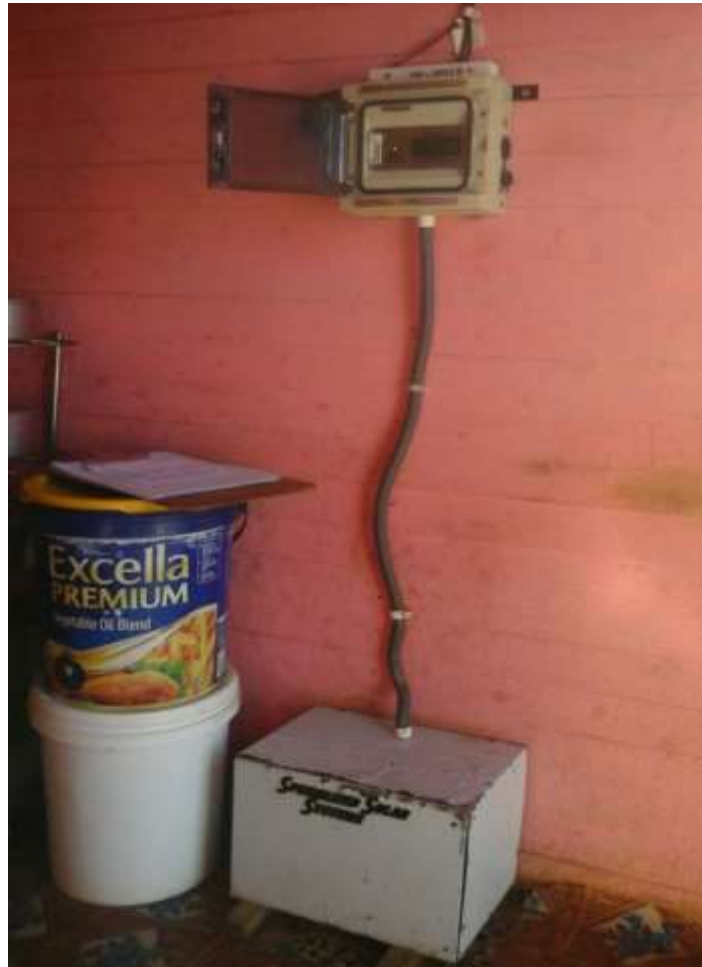
Figure 4.2: Installed Specialised Solar System
