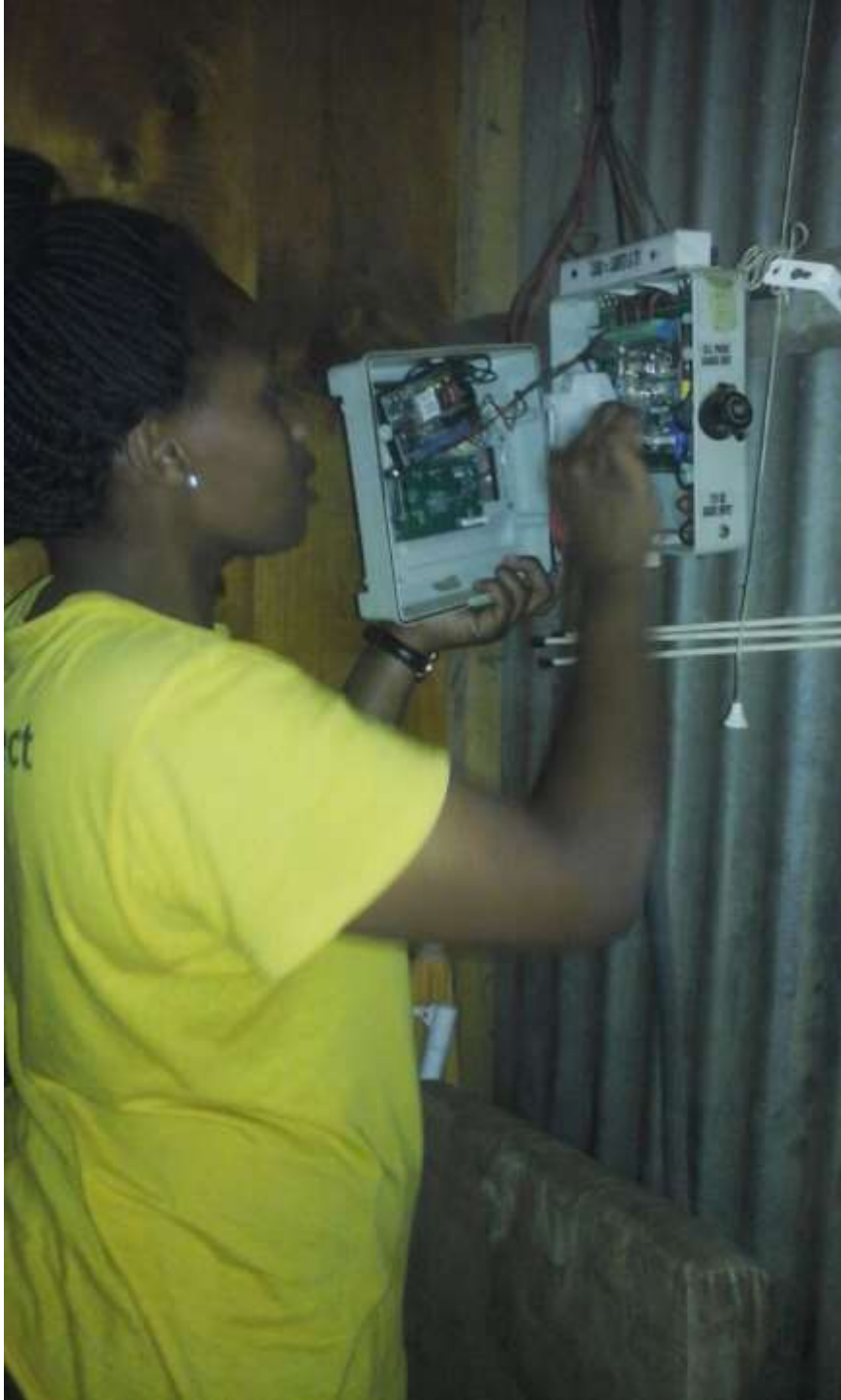
Figure 11: An iShack agent conducting maintenance checks on the Specialised Solar System
