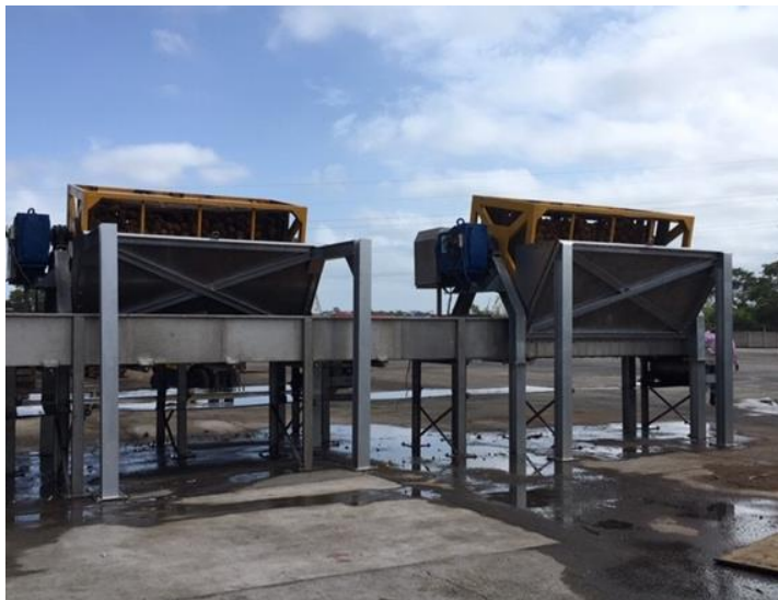
Figure 23 Facility 3013.17 replaced the 'dumper baths' with conveyor belts.
