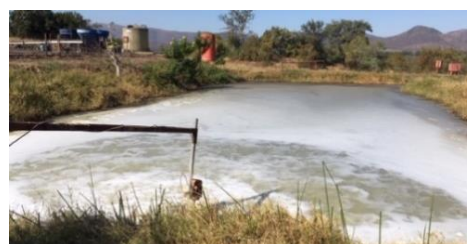
Figure 30 Aerobic lagoon at another facility with only one functioning aerator.
