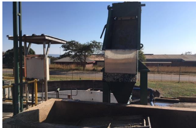
Figure 31 Static rundown screens were common at many facilities.
