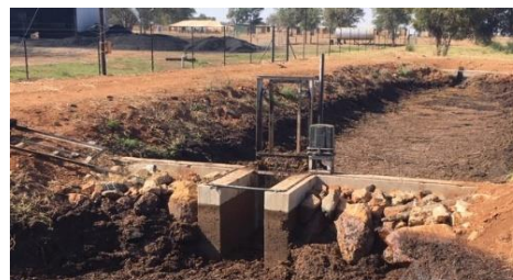
Figure 29 Rudimentary 'settlement dam' at one facility.
