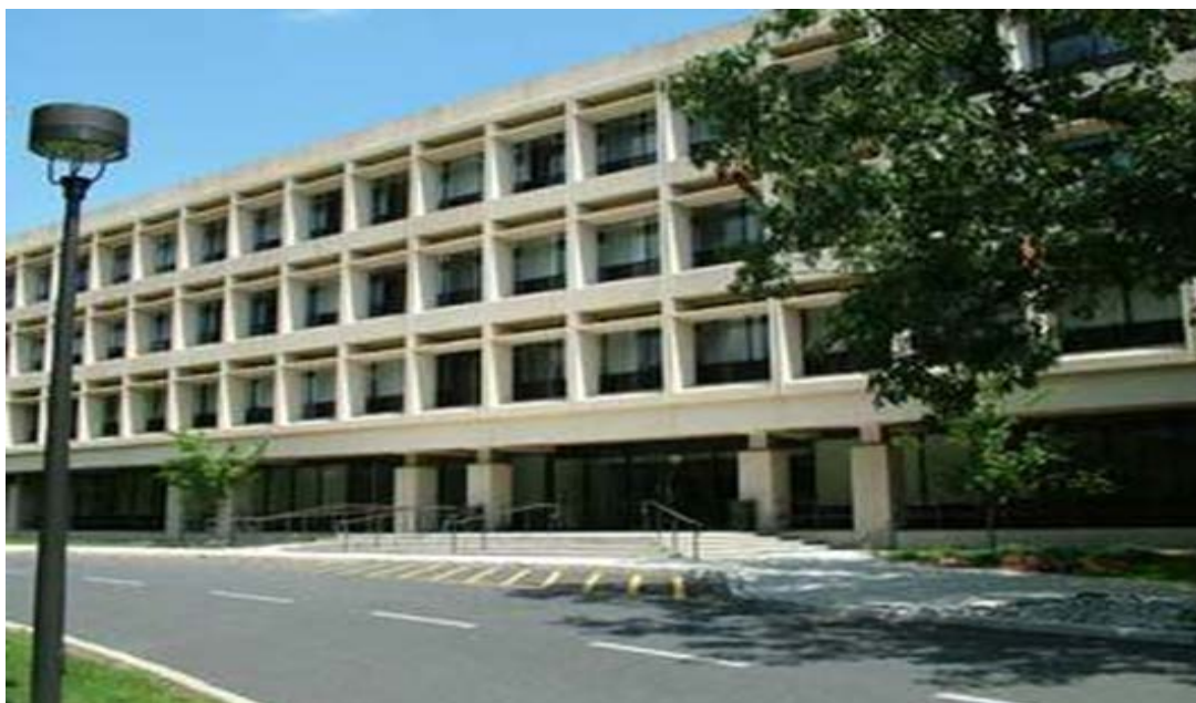
Figure 4.4: This is a photograph of a building that is similar to that of the selected schools.
