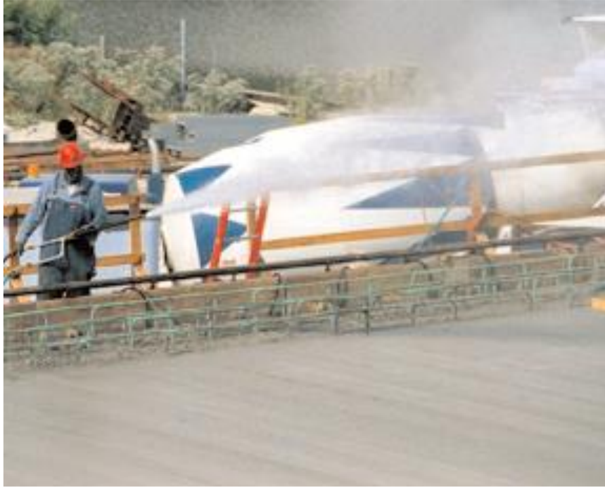
Figure 2.9: Misting of concrete (Kosmatka and Wilson, 2002)
