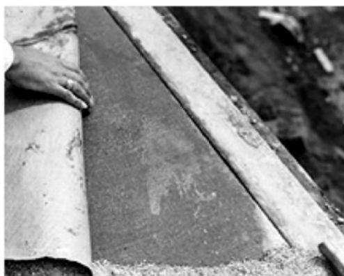
Figure 2.10: Impervious paper curing (Cement concrete & aggregate Australia, 2006)
