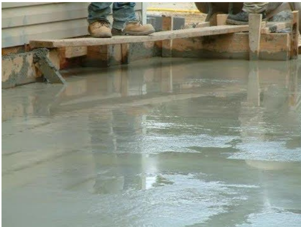
Figure 2.3: Bleeding of concrete ( https://www.youtube.com/user/WarunaThejana , 2018)
