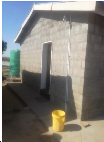
Photo 5: Block house with tank
