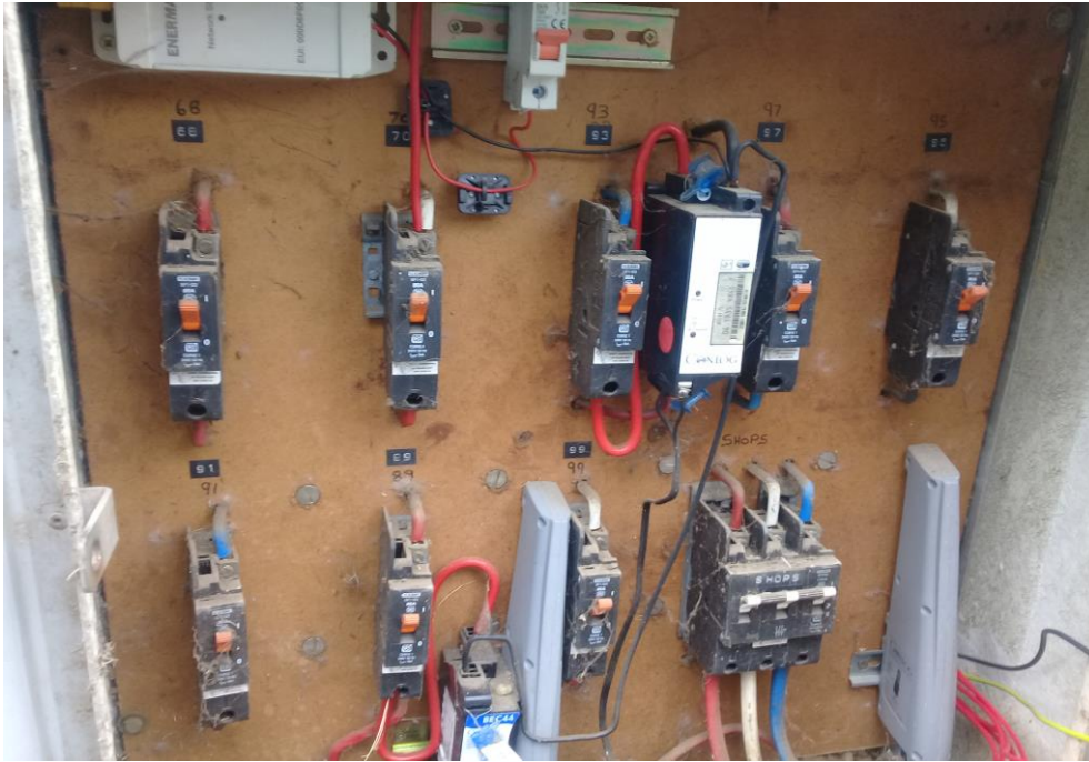
Figure 51: The customer supply side showing the lack of space to accommodate the current transformers.
