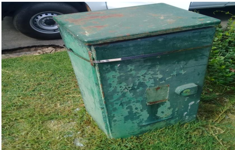
Figure 52: Old kiosks without enough space to accommodate the meters.
