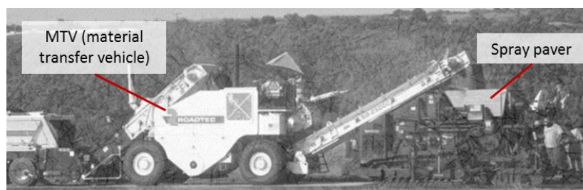
Figure 2.2.4.3b: Spray paver with material transfer vehicle (RoadTec, 2008)
