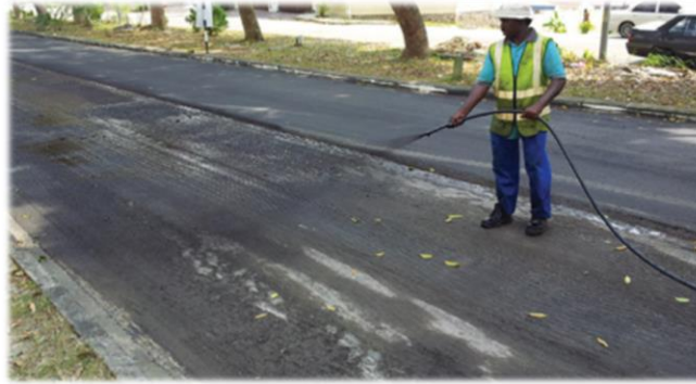
Figure 2.2.4.1b: Application of tack coat with hand sprayer (Yaacob et al., 2014)
