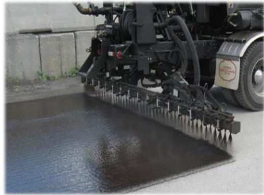
Figure 2.2.2.4a: Uniform tack coat coverage (RAHA Bitumen, 2016a)
