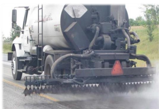
Tack coat distributor truck
