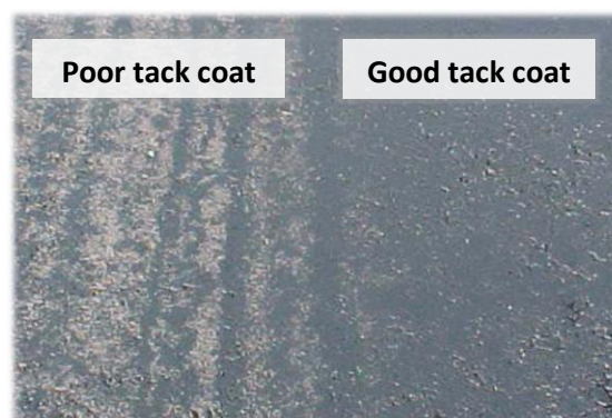
Figure 2.2.3.3a: Tack coat coverage (Federal Highway Administration, 2016)
