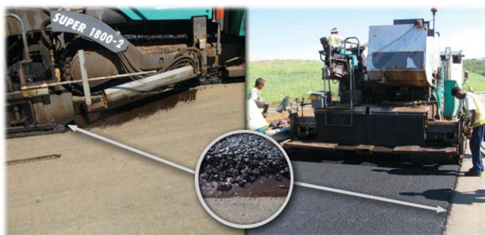
Figure 2.2.4d: Application of Elasto-Tack with spray paver (Tosas, 2019)
