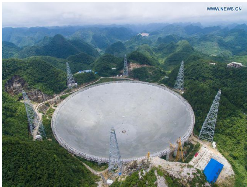
FIGURE 2.2: The world's largest single-aperture telescope, the Five-hundred-meter Aperture Spherical Telescope (FAST), was installed in 2016 in China [57].
