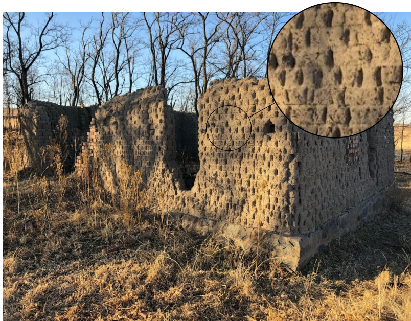
Figure 2.5: Eroded earth building near Kokstad in Kwazulu-Natal province, South Africa.
