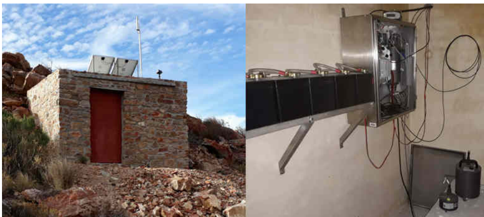
Figure 2.8: Outside (left) and inside (right) of the seismic vault at the main site area.
