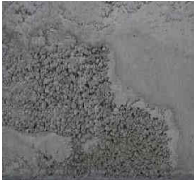
Figure 2.23: Concrete segregation due to high particle relative density coarse aggregate (Harikrishna, 2018).
