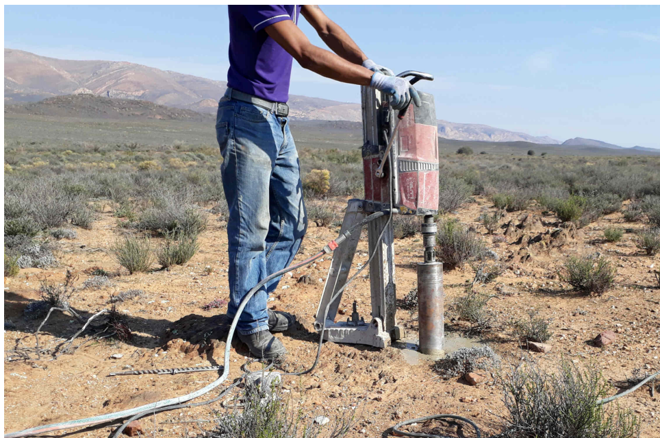
Figure 3.10: Drilling in progress.
