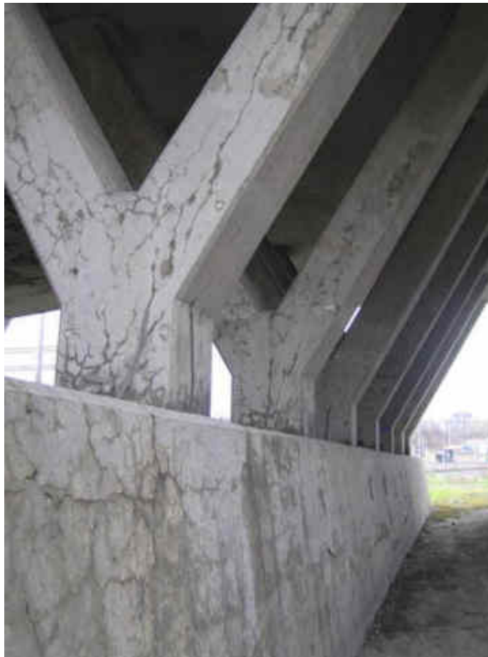
Figure 2.30: Du Vallon-Charest highway in Quebec, Canada, that was demolished due to ASR's (Fernandes and Broekmans, 2013).
