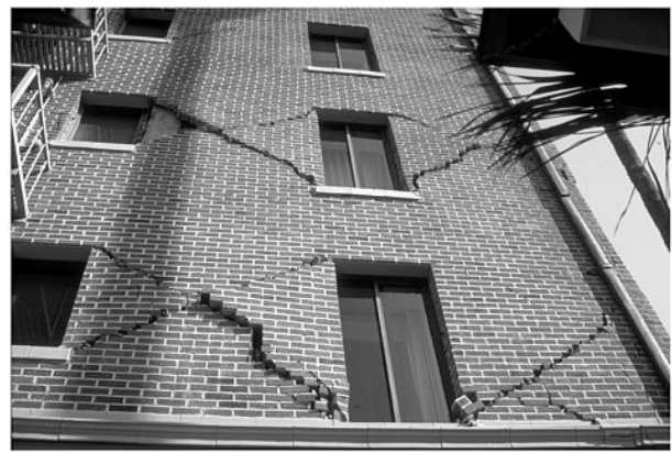
(b) Multi-storey building after an earthquake. (Council et al. , 2003)
