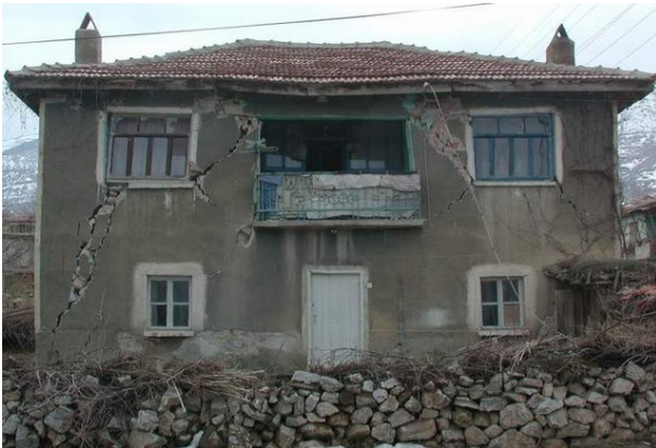
(a) Two storey masonry building after an earthquake (Churilov and Dumova-Jovanoska, 2011).
