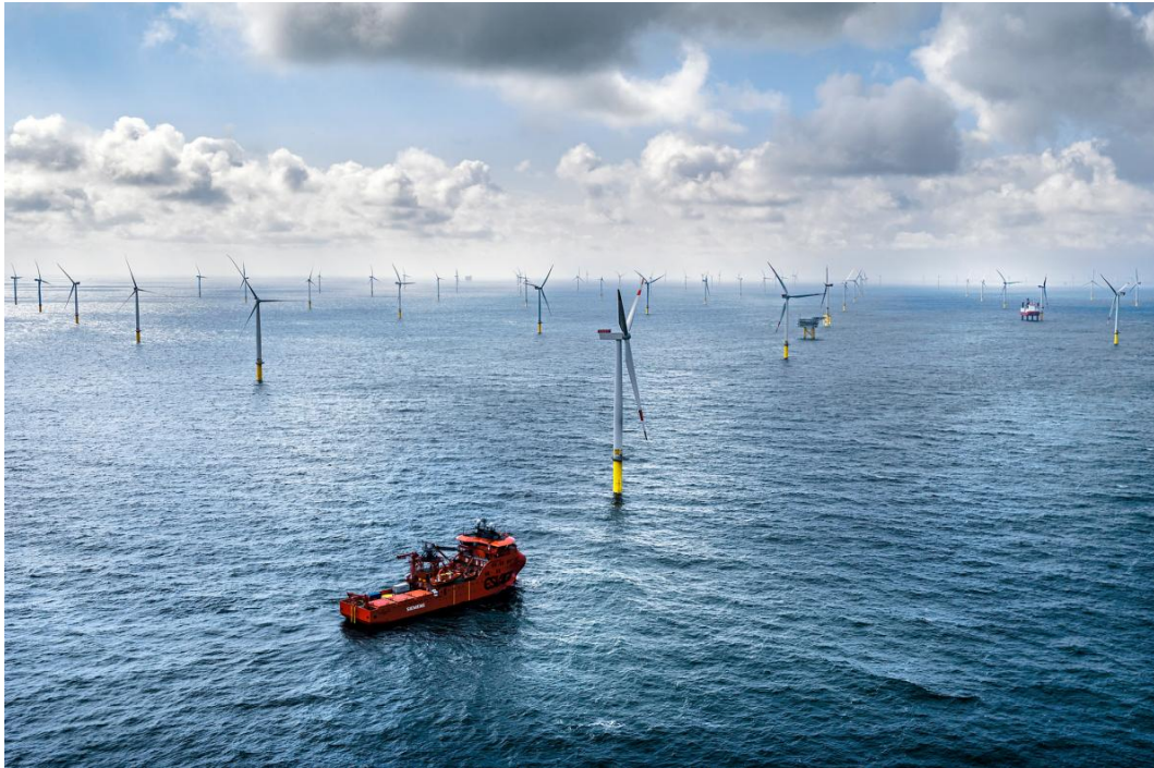
Figure 1.2: The Borkum Riffgrund 1 wind farm in the North Sea is part of the latest push for Germany’s Energiewende . It can produce enough power to supply 320 000 German households (Kunzig and Locatelli, 2015).
