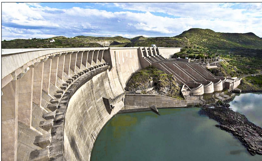
Figure 1 Roberts splitters on the Vanderkloof Dam spillway (vanderkloofd.com 2014)
