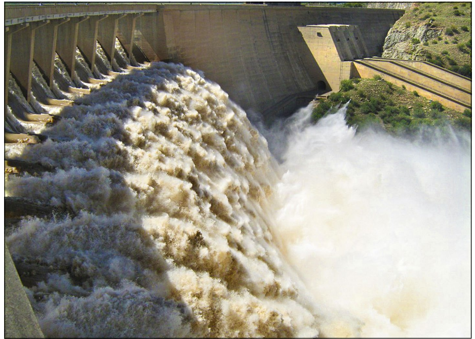
Figure 2 Roberts splitters in operation on the Gariep Dam spillway (Calitz & Basson 2015)
