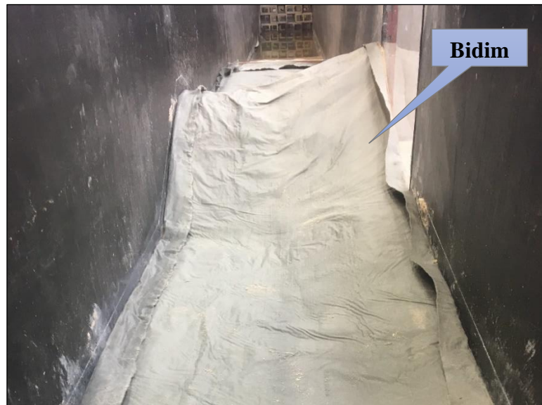
Figure 20: The Bidim geotextile filter layer placed on top of the gravel
