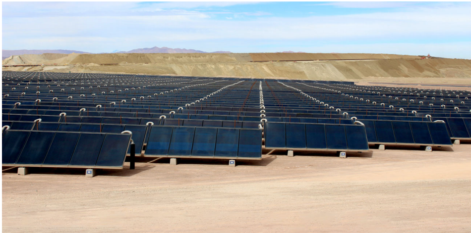
Figure 1.1: Pampa Elvira SPH plant, Chile. Picture: Arcon-Sunmark (2017)
