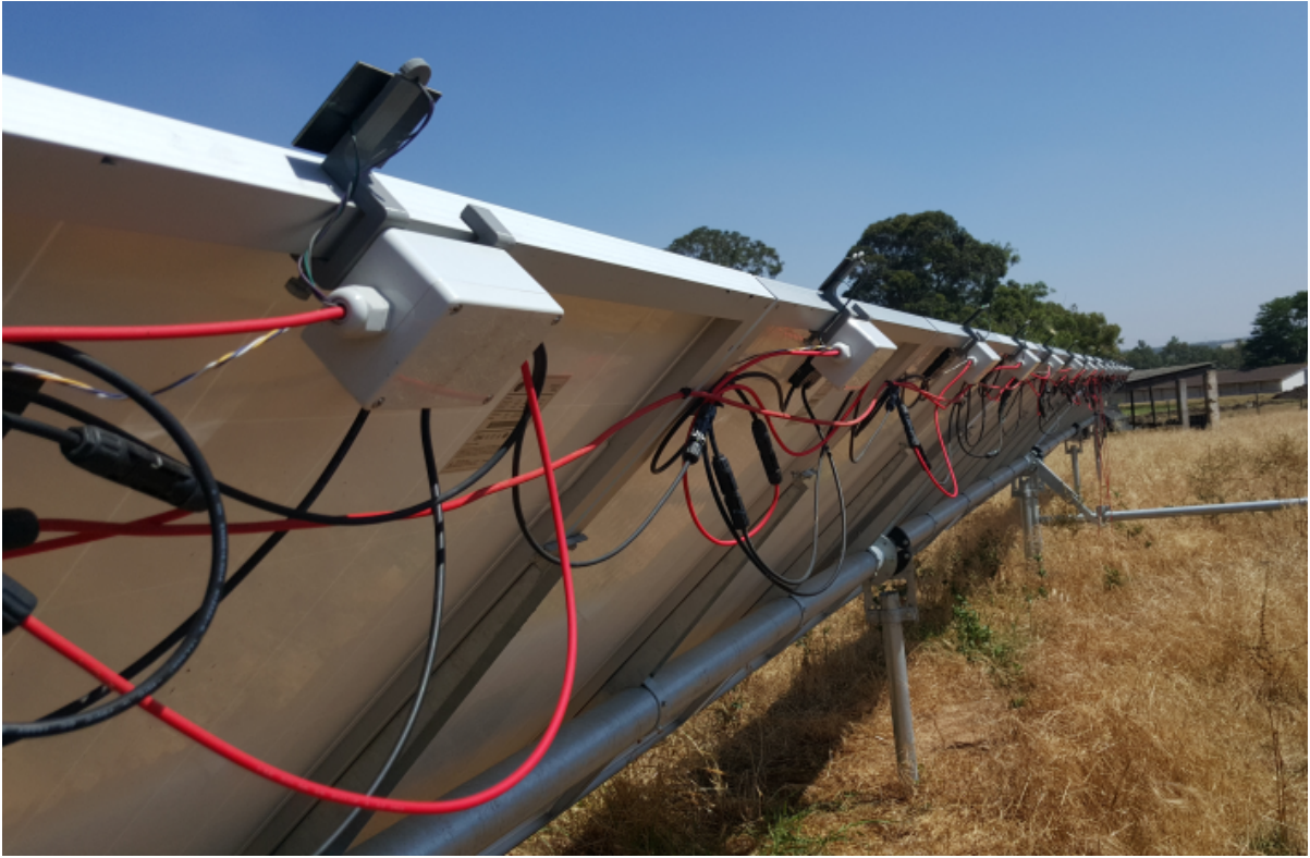
Figure 6.23: Sensor Node Side-Bottom View PV Plant Field Test
