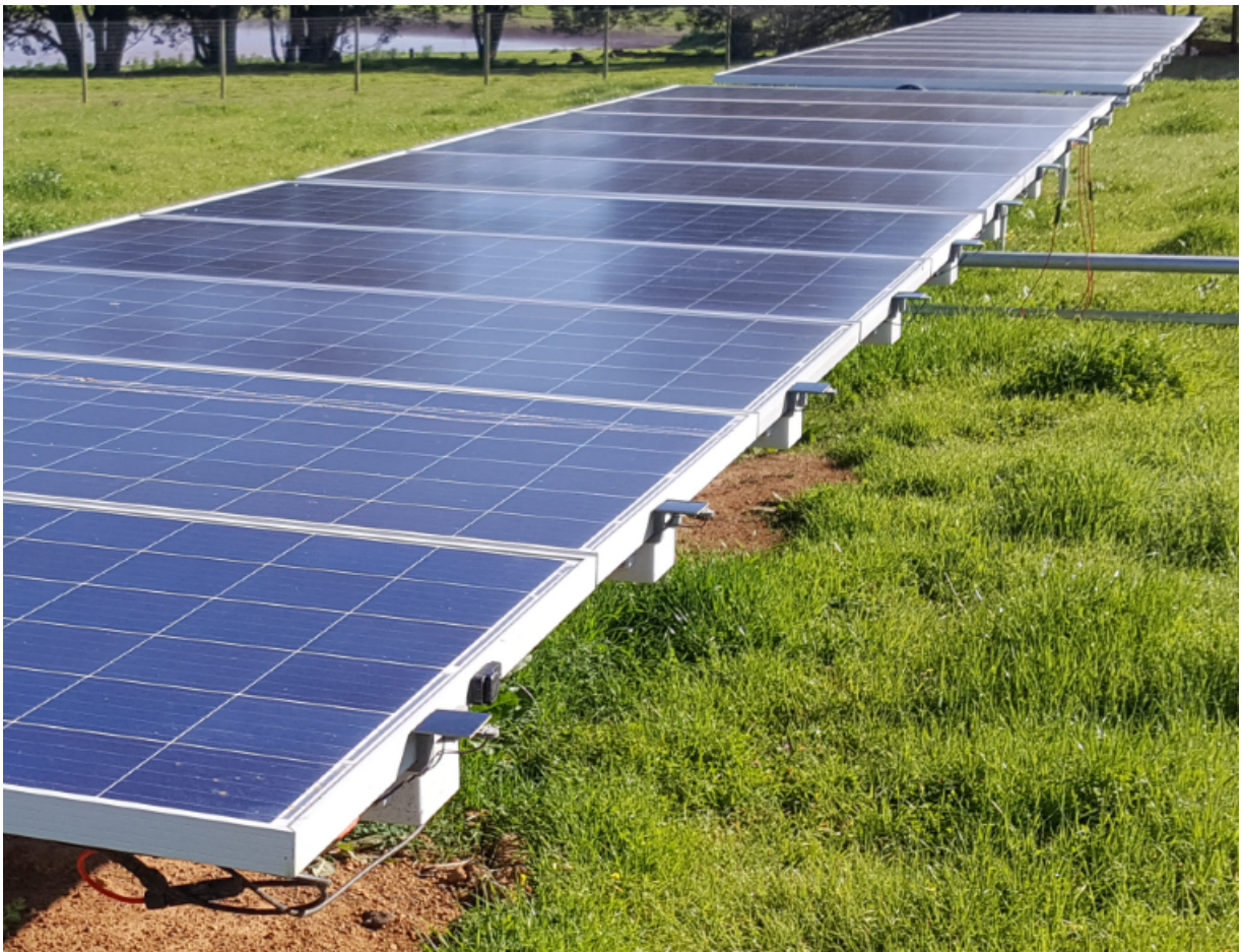
Figure 6.24: Sensor Node Side-Top View PV Plant Field Test
