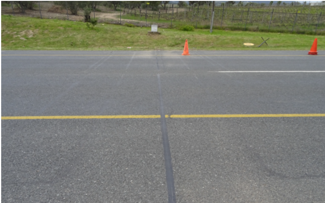
Figure 3.7: Side view of the R44 Traffic Count Station
