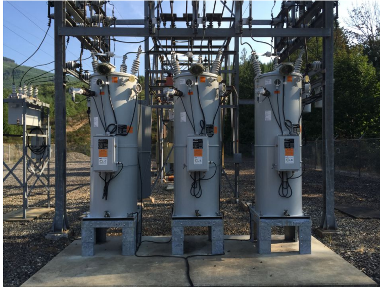
Figure 3.11: Distribution Substation Voltage Regulators [29]
