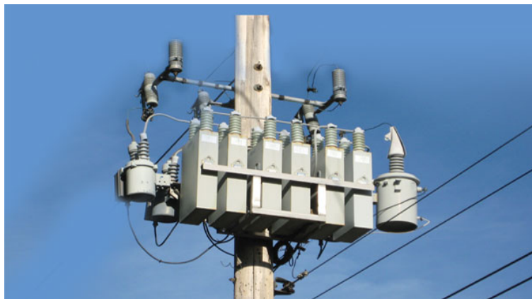
Figure 3.12: Shunt Capacitor Bank [30]
