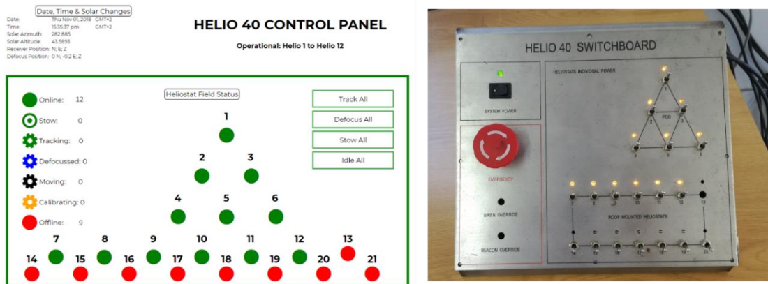
Figure 37: Control panel on the left showing heliostats connected to the Control panel, and the switch board indicating the heliostats are powered with the LEDs.
