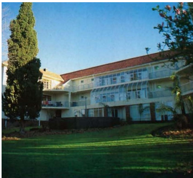
Figure 4: The Residence Huis de Villiers Following its renovation in 1996
