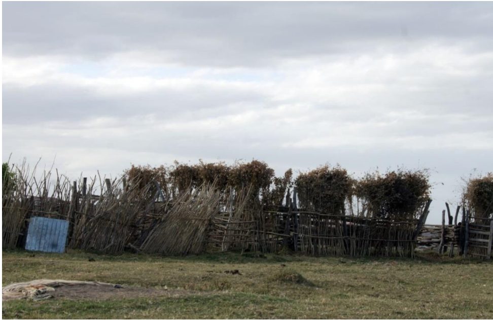
Figure 6.2 The photo above shows the kraal constructed as is historically done, with organic, lush, green materials and wood found in the valleys.
