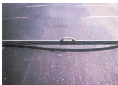
Figure 2.8: Severe form of rutting (TMH 9, 1992)
