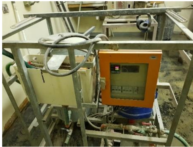
Figure 3.25: Water Heating Unit (WHU)
