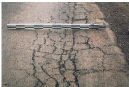
Figure 2.9: Crocodile cracking due to fatigue (TMH 9, 1992)
