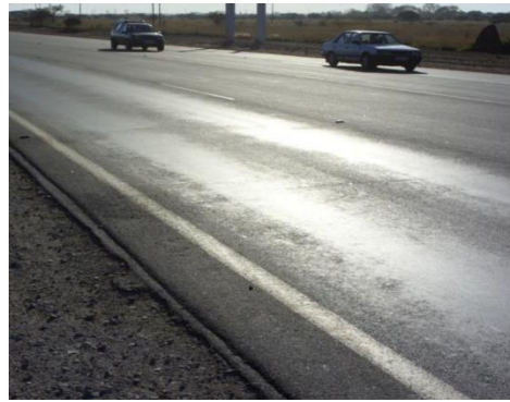
Figure 2.7: Asphalt with poor skid resistance (SAPEM Chapter 9, 2014)
