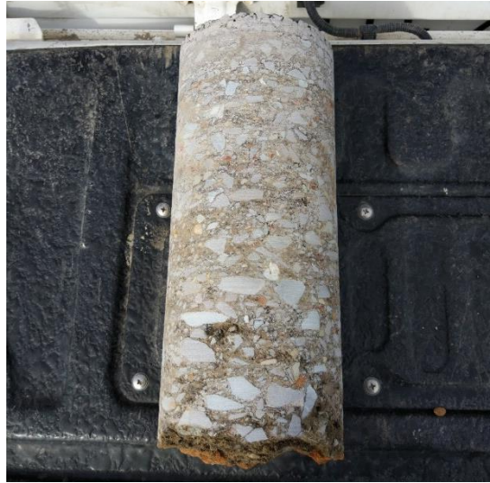
Figure 3.6: Asphalt and BSM layer
