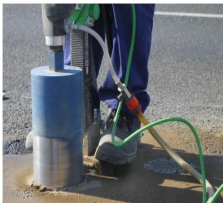
Figure 3.5: Core drill operation
