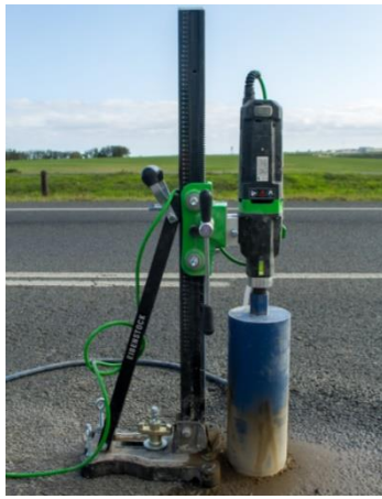
Figure 3.4: Core drill setup
