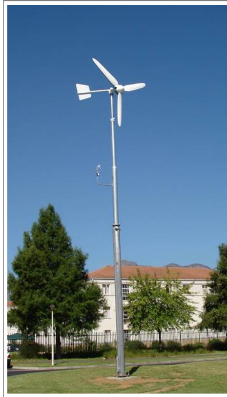
Figure 1.9: Small-scale wind turbine at Stellenbosch University.
