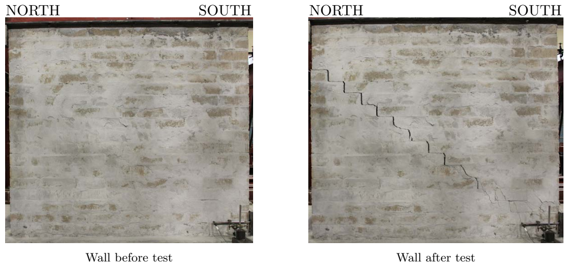
Figure 5.15: Second Mock Wall Test
