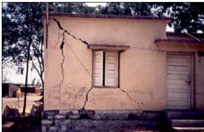
Figure 2.6: Cracks in an Unreinforced Brick Masonry Building( Bhattacharya et al., 2014 )
