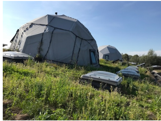
Photo 4.20. Recycled tyres for the back wall of the Earthship & Photo 4.21. Kite shape structure of the domes (Source: Sharné Bloem)
