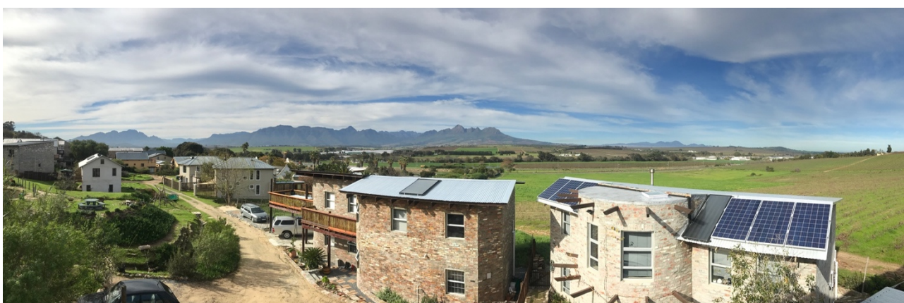
Photo 1.2. Lynedoch EcoVillage view on some micro-grid panels (source: Sharné Bloem).
