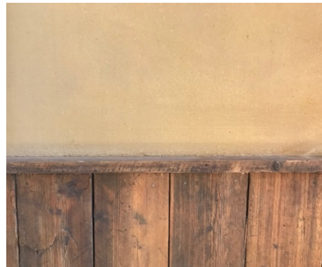
Photo 4.22. Recycled pallets timber as a ceiling & Photo 4.23. Recycled scaffolding timber as wall cladding (Source: Sharné Bloem)
