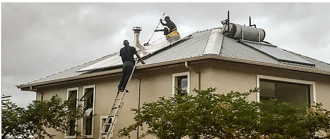
Photo 4.33. PV panels being cleaned (Source: Sharné Bloem).
