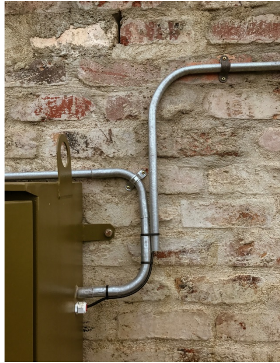
Photo 4.31. IP65 Box (Source: Sharné Bloem) & Photo 4.32. DC Conduits (Source: Sharné Bloem).
