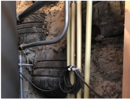
Photo 4.20. Recycled tyres for the back wall of the Earthship & Photo 4.21. Kite shape structure of the domes (Source: Sharné Bloem)
