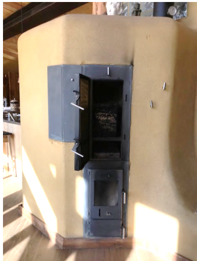
Photo 4.24. Rocket mass heating system & Photo 4.25. Feeding and burning chambers (Source: Sharné Bloem)
