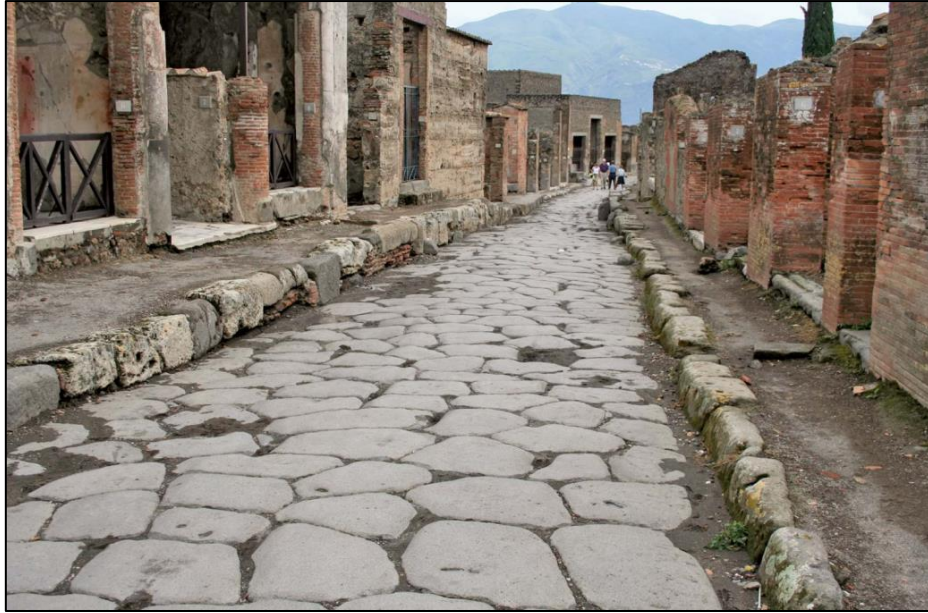
Figure 7: Carriageway with elevated sidewalks in Pompeii, Ancient Roman City (Huxham, 2014)
