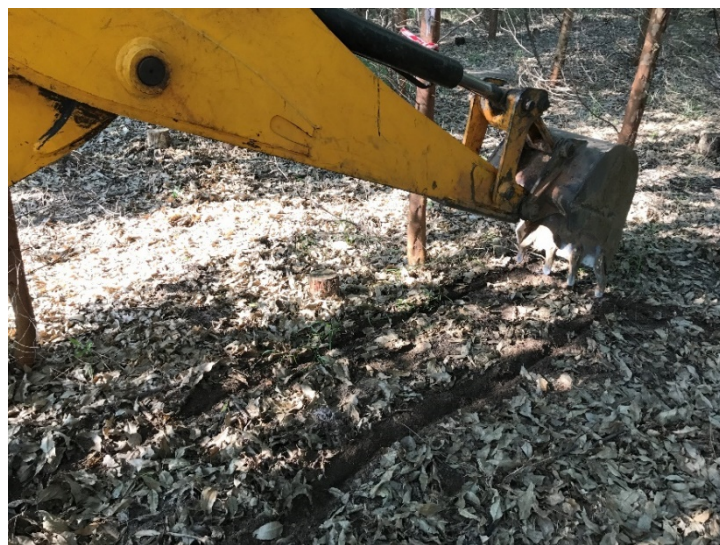
Figure 3.5: Mechanical digger opening up a trench to expose the root system.
