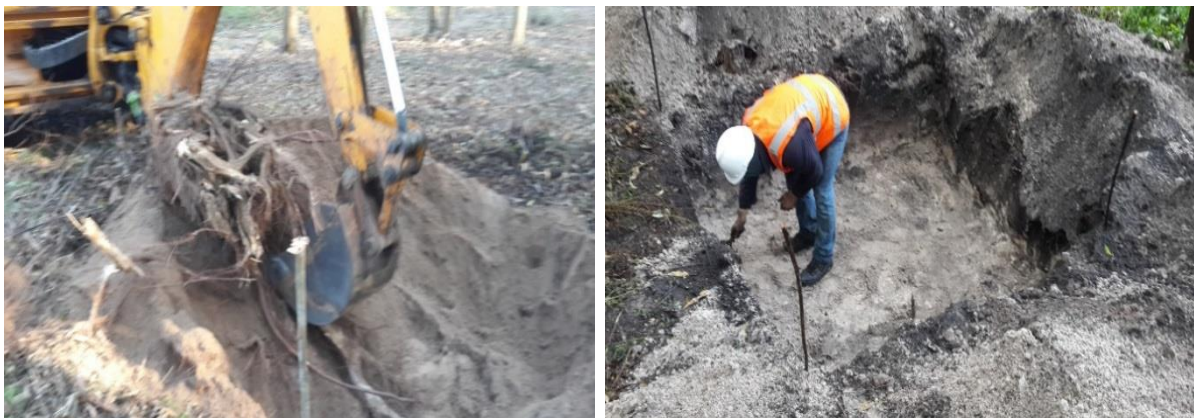
Figure 3.4: The bulk of the root bole was excavated using a back-actor, after which the hole was further excavated by hand for more precise digging.
