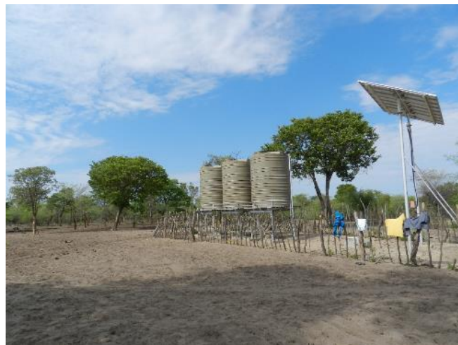
Communal water point
