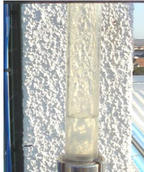
Figure 12 Right-hand side vertical pipe sight glass indicating annular flow
