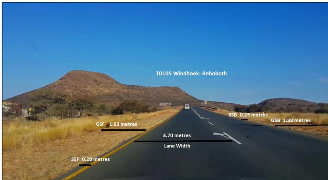
Figure 4.22 Road Section T0105
