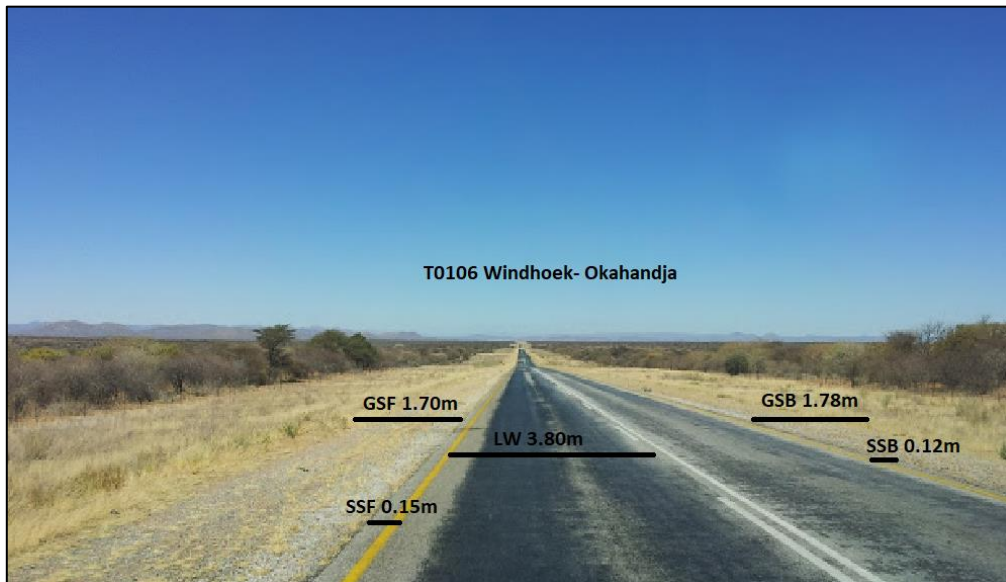
Figure 4.12 Road Section T0106
