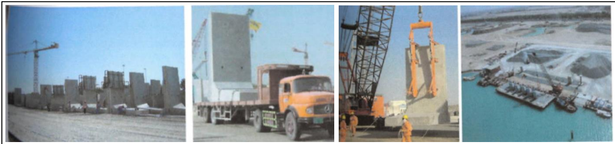
Figure 2-11: Casting and placement of L-elements at Al Raha, Western precinct (Wehr, Freitag and Kohler, 2015)
