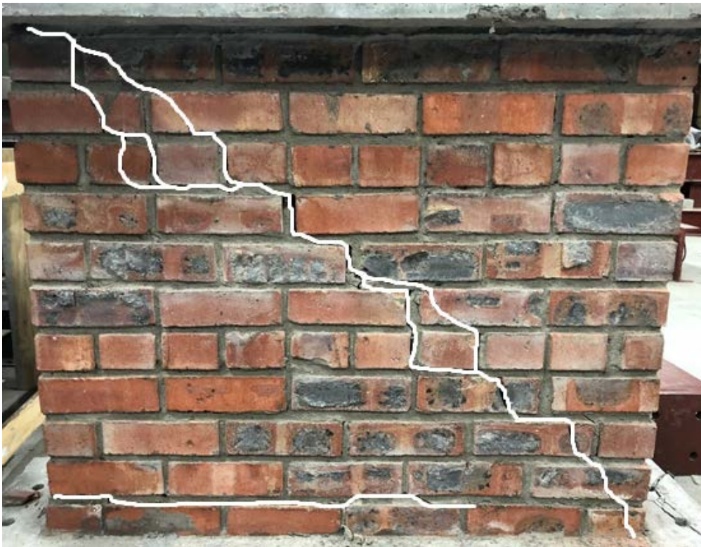
Figure 5.17: SW-100-200-02 crack pattern in the masonry.
