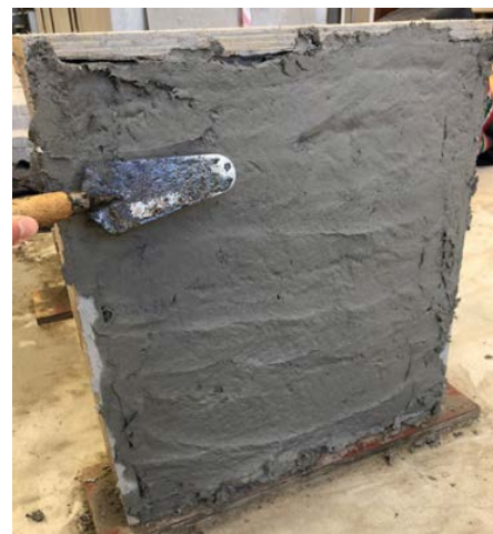
(d) Near completion of trowelling
