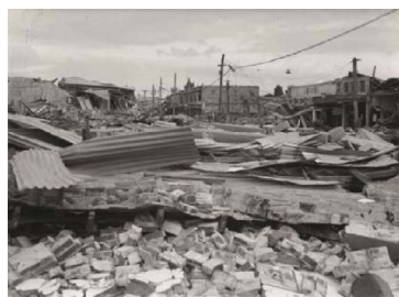
a) Damage caused by the 1931 M7.8 Hawke's Bay earthquake
