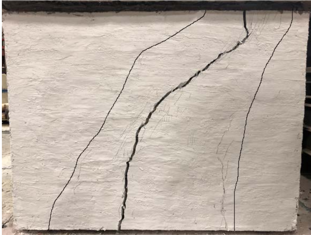
Figure 5.18: SW-100-200-02 crack patterns outlined.
