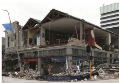
b) Collapse of out-of-plane loaded URM walls in the 2010 M7.1 Darfield earthquake
