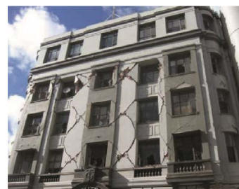
c) In-plane diagonal cracks caused by the 2011 M6.3 Christchurch earthquake
