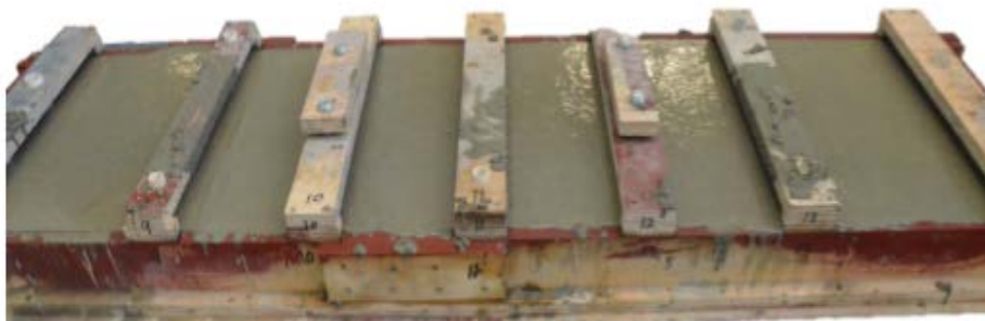
(b) Beam casted with SCC
