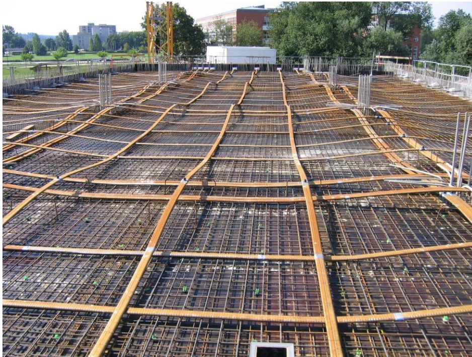
Figure 3.6: Post-tensioned slab prior to concrete pouring (Post-tensioning, n.d.)
