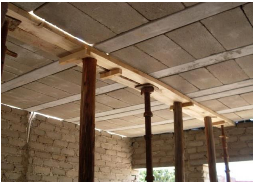
Figure 3.10: Propping of a conventional Rib and Block system (Nyati Slabs South Africa: Rib and block propping, n.d.)
