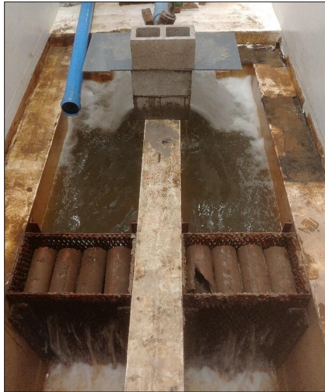
Figure B.5 Settling basin used to trap outflowing sediment
