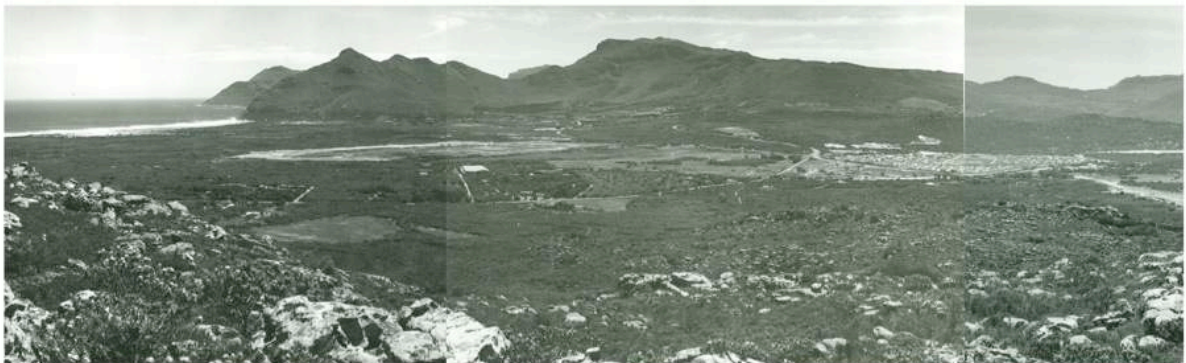
Photo 4.2: Historical view of the Noordhoek valley looking north towards the Chapmans Peak Mountains taken in 1974. Source: Cape Archives Depot, CA Photo Collection. (CA1648, CA1651, CA1652)
