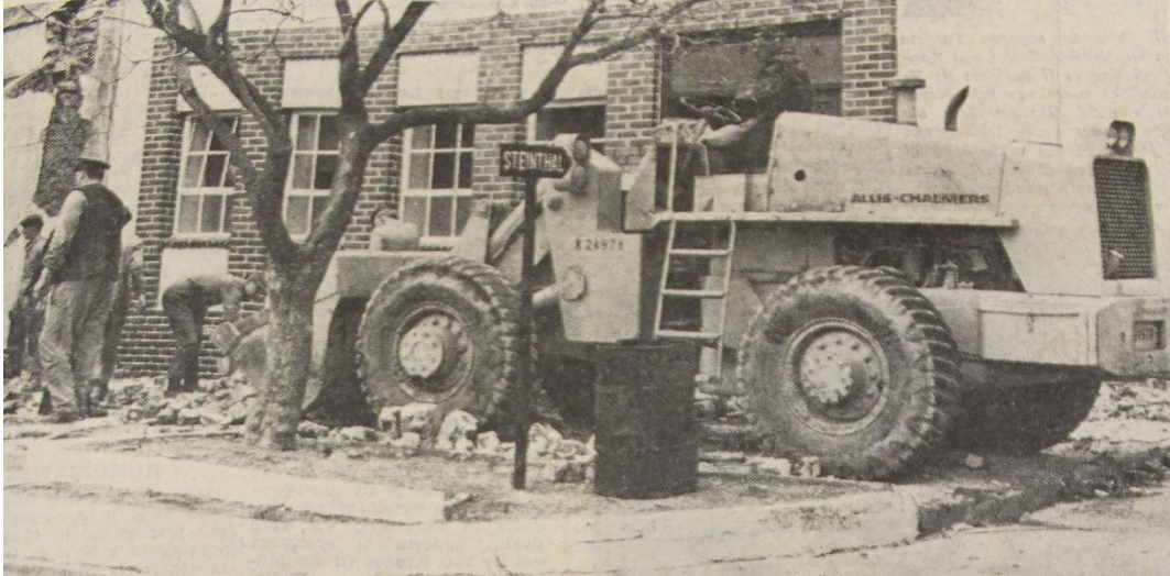
FIGURE 2.6: The wet weather aggravated the condition of the earthquake-damaged buildings, as the rain softened the exposed bricks. The above illustration is the demolition operation of the bank situated in the main road of Tulbagh. 155
