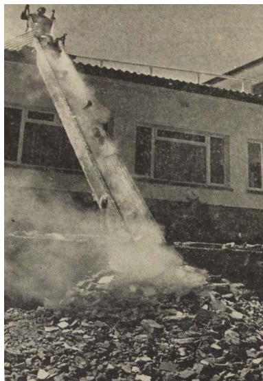
FIGURE 3.5: The Belmont Hotel in Ceres was severely damaged by the earthquake, and was in dire need of repair. 387
