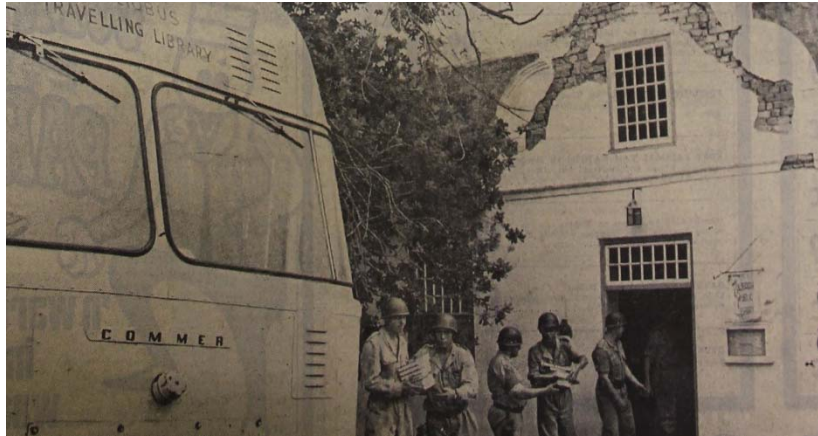
FIGURE 3.2: The army helped clear all the books from the Tulbagh Library, as the building was severely damaged by the earthquake. The books were transported to the main library in Cape Town. 290
