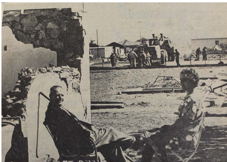
FIGURE 3.4: Demolition in Wolseley 378
